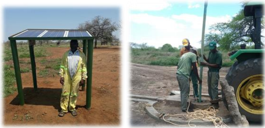
Fig.9 - Solar panel installation and borehole being fixed.
